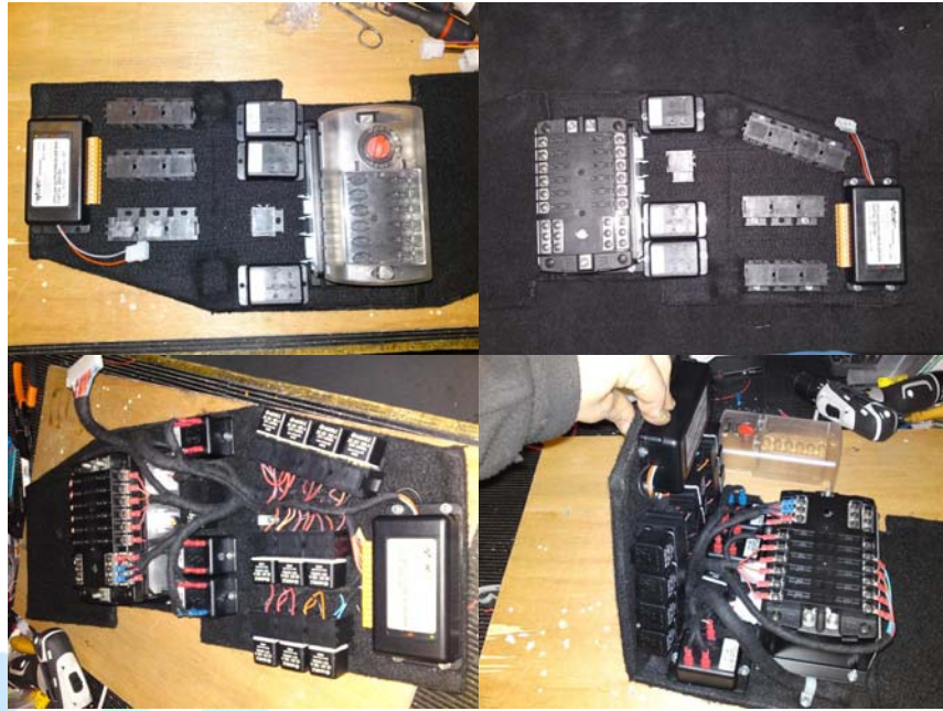
Figure 7,8,9 & 10 Discovery Lights/Sirens Control Relays Etc
